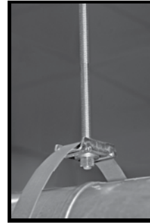
Spiral Buckle with threaded rod
