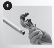
Cut tubing and remove PE coating to expose a minimum of 4 corrugations.
