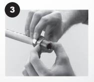
Slide nut over retainer ring and hand tighten.
