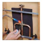
*The Insurance Pad* is the ultimate heat shield. Use wet or dry, where higher temperature protection and prolonged use is required. Great for use with
