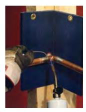
The Torch-Guard<sup>®</sup> Heat Shield provides protection up to, but not exceeding 2500°F. It is asbestos free and features
