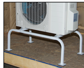
Photo #2 (On left) Mini-Split 12" Stand (side view) showing connection to stand.
