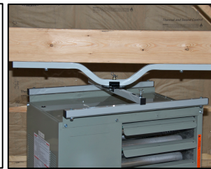
Photo #2 (On left) H-Brackets, Spreader Arm and Circular Adj. Plate attached to Unit Heater.
