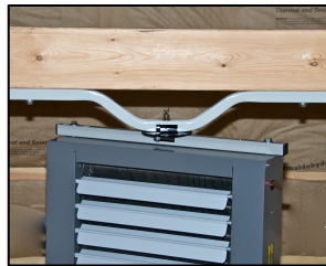
Photo #2 (On left) Spreader Arm and Circular Adjustment Plate attached to Unit Heater.
