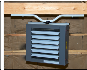
Photo #2 (On left) Spreader Arm and Circular Adjustment Plate attached to Unit Heater.
