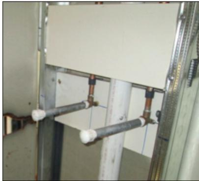
system and a PVC threaded cap is used to seal the nipple as shown in the photograph.
