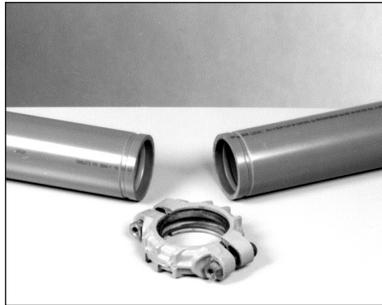
2. Check the pipe ends for any damage, roll marks, projections, or indentations on the outside surface between the groove and the end of the pipe. This is the sealing area, and it must be free of any defects.
