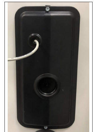
Figure 17 - Access Panel Reinstalled
