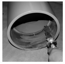
• **NOTICE:** Pipe diameters 6" and larger must be installed using IPS P-70 or Oatey Industrial Grade primers.
