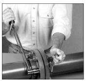
When installing flanges in a buried application where 8. settling could occur, the flange must be supported to maintain proper alignment in service.
