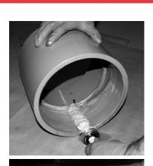
Apply a second full coat of cement to the pipe surface aggressively working it in.
