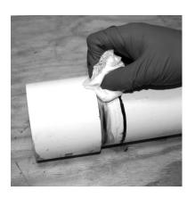
• Align all piping system components properly without strain. Do not bend or pull pipe into position after being solvent welded.
