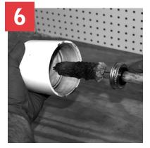
Apply primer to the pipe surface to a point ½" beyond the hub depth. Aggressively work the primer into the surface.
