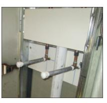
system and a PVC threaded cap is used to seal the nipple as shown in the photograph.
