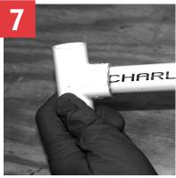
Insert pipe into fitting hub giving
