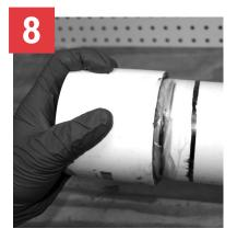
Insert pipe into the fitting hub
