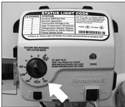
Figure 40 - Turn gas control/temperature knob OFF.
