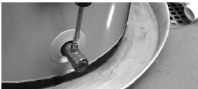
Figure 42 - Draining the water heater.
