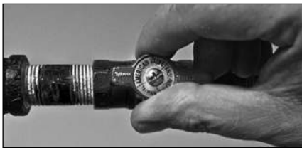
Figure 32 - Gas valve in "on" position
