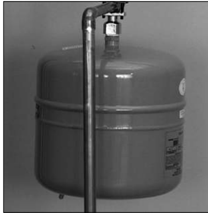
Figure 29 - The Thermal Expansion Tank should be pressurized with air, using a hand pump, to match the home's incoming water pressure.
