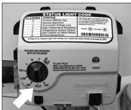
Figure 48 - Gas control/valve.
