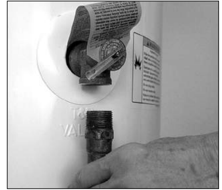
Figure 21 - Removing the T&P Relief Valve discharge pipe.
