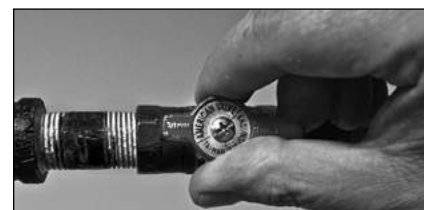
Figure 58 - Gas valve in “on” position.
