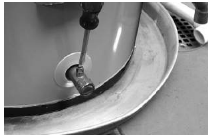
Figure 20 - Draining the old water heater.
