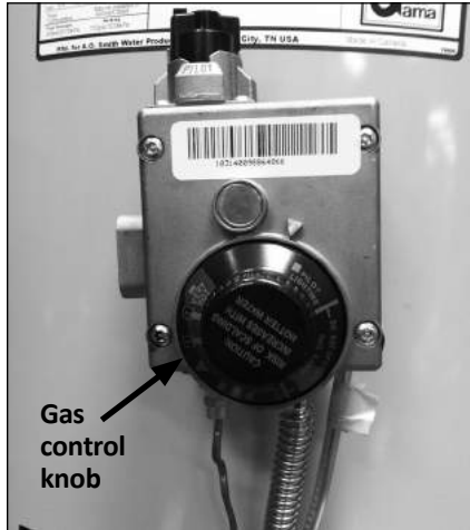
Figure 17 - Turn gas control/temperature knob OFF.
