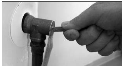
Figure 45 - T&P Relief Valve.
