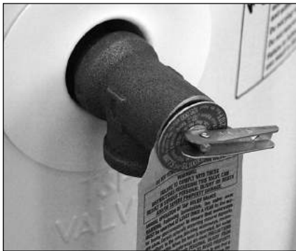
Figure 25 - Temperature and Pressure Relief Valve
