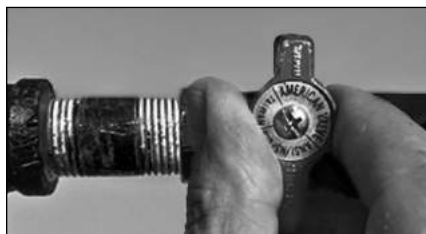
Figure 50 - Gas valve in “off” position.
