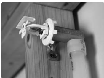
Figure 1-4: ProPEX Elbow with HSW Sprinkler Head
