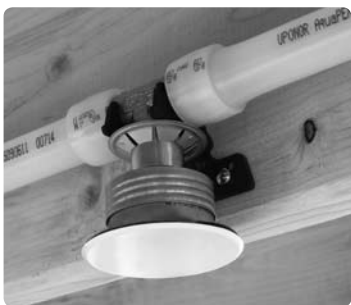
Figure 1-3: ProPEX Tee with RFC Sprinkler Head
