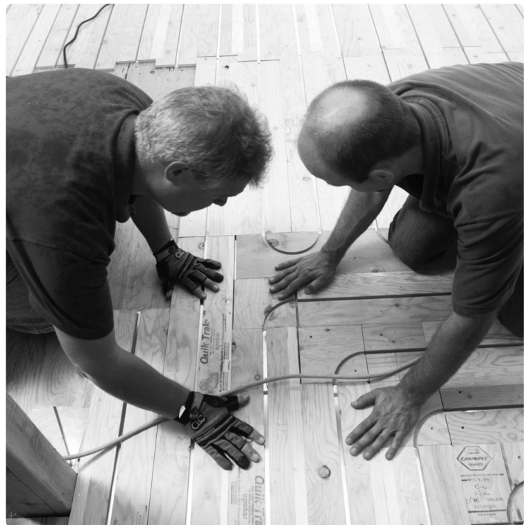
Figure 4: Installing Quik Trak Panels
