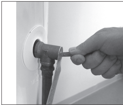
Figure 51 - T&P Relief Valve.
