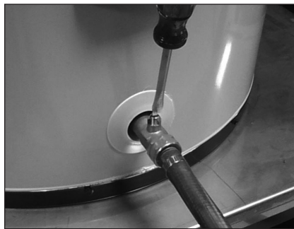
Figure 11 - Draining the old water heater.
