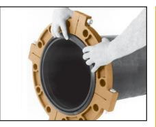
**INSTALL GASKET**—Check the gasket grade to verify that it is properly suited for the intended service. Lubricate the entire surface of the gasket and the flange cavity using the appropriate Gruvlok Lubricant. Place the Gruvlok Flange Gasket around the pipe end by pressing the gasket into the cavity between the pipe O.D. and flange recess. Move around the gasket in both directions until the gasket is fully seated in the flange gasket cavity.
