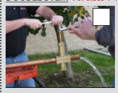
This is a TWO person operation. Use a 9/16" socket wrench on the stem cutter, and with the help of a second person, use an open end wrench on the outer stem. This sets the depth of the cut and prevents the cutter from binding. Slowly turn both wrenches at the same time.
