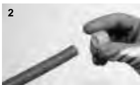
Figure 6: Place the ProPEX ring over the end of the pipe.
