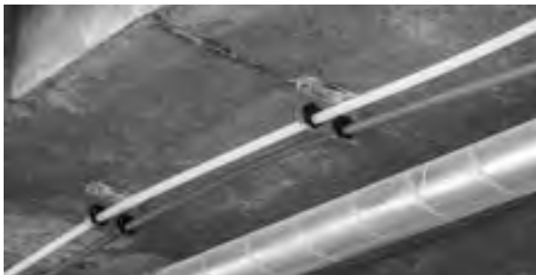
Figure 24: Supporting small-diameter coiled PEX
