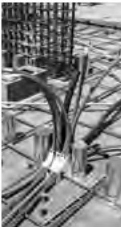
Figure 55: In-slab installation
