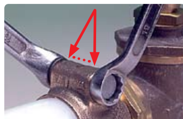
Figure 4-33: Grip and Seal Between Fitting and Pipe
