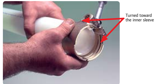
Figure 4-29: Mount the Outer Sleeve
