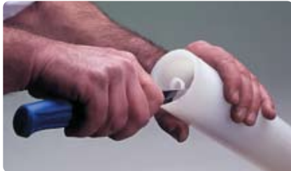
Figure 4-25: Chamfering
