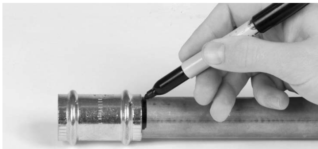
Figure 9 – Marking the Tubing After Fully Inserting Tube
