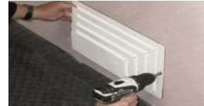
ATTACH GRILLE TO WALL WITH PROVIDED SCREWS.
