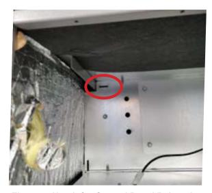
Figure 5. Notch for Control Panel Relocation
