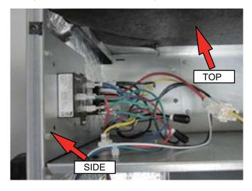
Figure 4. Electrical Connections (Upflow Configuration)
