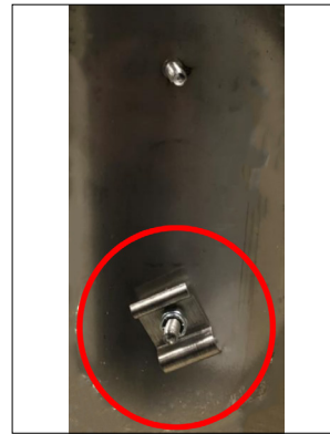
Figure 12 - Sensor Clip Installed on the Lower Stud
