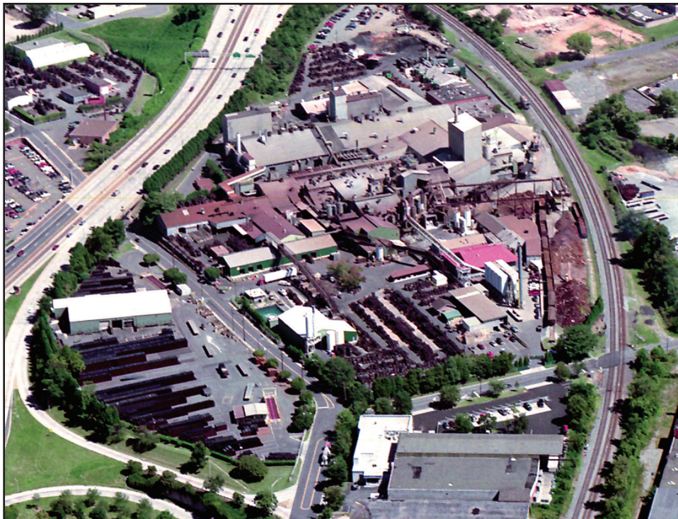
Charlotte Pipe and Foundry Company, Cast Iron Division
