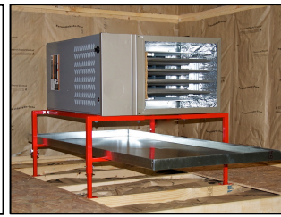
Photo #2 (On left) Quick Stand assembled in place with Secondary Drain Pan.
