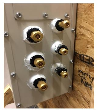
13. Complete all line set and electrical connections as required by branch box manufacturer.
