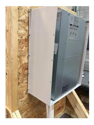
8. Complete all wiring and piping to branch box at this point. Refer to Branch Box installation instructions for Dip switch settings and addressing.
