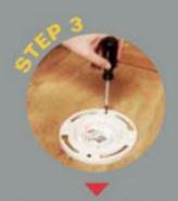
Secure toilet flange to floor with fasteners.
