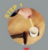
Cut pipe to fit inside of toilet flange.
