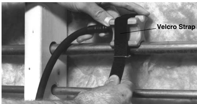
Figure 5 – Applying Freeze Head with Velcro Strap
