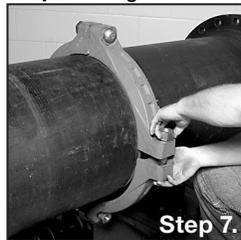
**Step 7.** Bring the next section of the housing into position. Insert a bolt into the coupling and finger tighten the nut.
