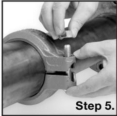
**Step 5.** Insert the other bolt and nut into the coupling and rotate both nuts until finger tight. Verify that the bolt heads are fully recessed in the housing.
