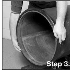
**Step 3.** Install the gasket by placing it over the end of the first pipe section. For larger pipe diameters, it may be easier to roll the gasket inside out, then on to the pipe end.
