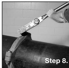
**Step 8.** Tighten nuts uniformly to the recommended bolt torque per Table A.
