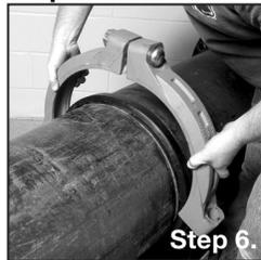
**Step 6.** Assemble two sections of the housing by inserting a bolt into the coupling and loosely engaging the nut. (For four segment couplings it may be easier to assemble two halves first.)
