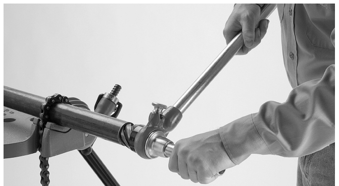
Figure 4 – Reaming End Of Pipe
