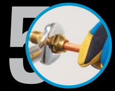
Thread the flare nut onto the male fitting and tighten using correct tools to equipment manufacturer torque specifications.
