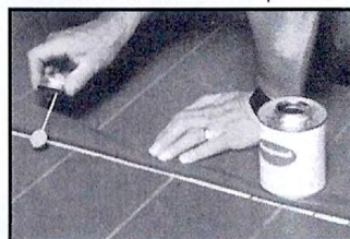
3 Weld both sides of seams with Flexible PVC Cement
