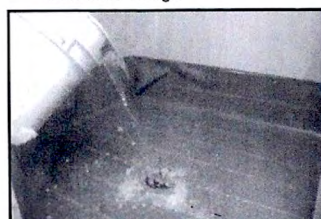
13 Bolt on top half of drain, plug drain, and water test
