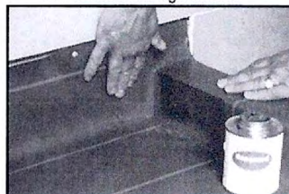
9 Weld Pre-formed corners/curb protectors in place
