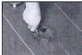
10 Carefully trim pan to expose drain
