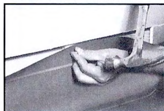
5 Nail (or screw) pan to studs or blocking
