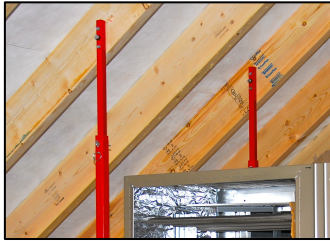
Photo #1 (On left) Extension Arms mounted to Rafters with enclosed hardware.
