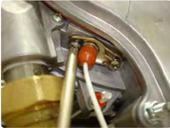
Figure 142 Removal of Ignition electrode
