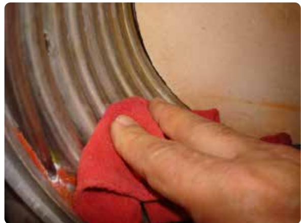
Figure 152 Cleaning the heat exchanger
