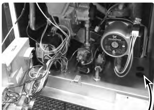
Figure 65 Thermostat or sensor wiring entrances
