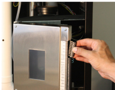
Line voltage load pump terminals
