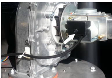
Gas valve electrical connector
