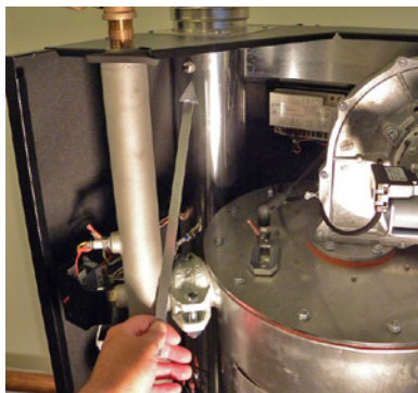
Flue gas test port plug
