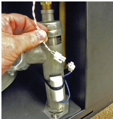
Return water temperature sensor
