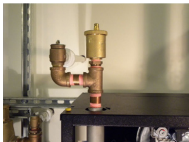
Relief valve and air vent assembly (recommended configuration)
