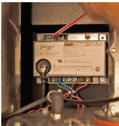
Fenwal ignition module - Microamp ( \mu A) test points are shown at top left corner of module (beside red L.E.D.)
