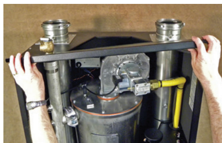
Lift top cover up at front
