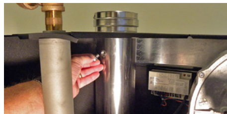
Removal of flue gas test port plug
