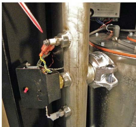
Low Water Cut-Off Probe on Supply Riser
