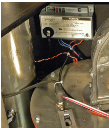
Ignitor Cable connected to Ignitor
