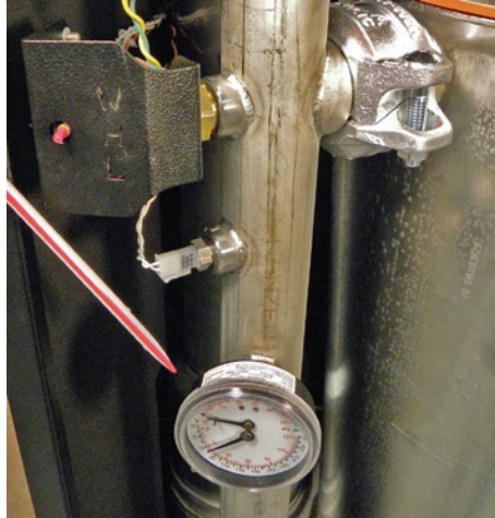
Tridicator Gauge on Supply Riser
