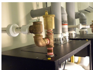
Relief valve and air vent assembly (relief valve discharge piping - required by code - piped to back)
