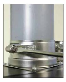
For PPs material, use the transition / adaptor fitting (Sch 40 to PPs) offered by the respective PPs manufacturers Centrotherm / Innoflue™ (their part # ISAA0303 or # ISAA0404) or M&G Dura Vent / PolyPro™ (# 3PPs-AD), (# 4PPs-AD) or Z-Flex/Z\_DENS (# 2ZDCPVCG3). For PPs material exposed to outdoor weather, follow the venting supplier's recommendations on UV protection.
