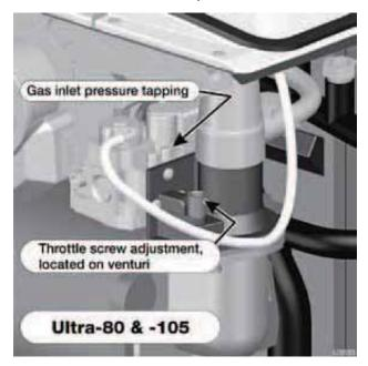
Figure 38 Models 155, 230 & 299 — Throttle screw location (ONLY for use by a qualified technician, using calibrated combustion test instruments)
