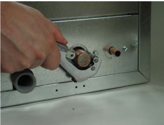
Cut end of connection as shown.
