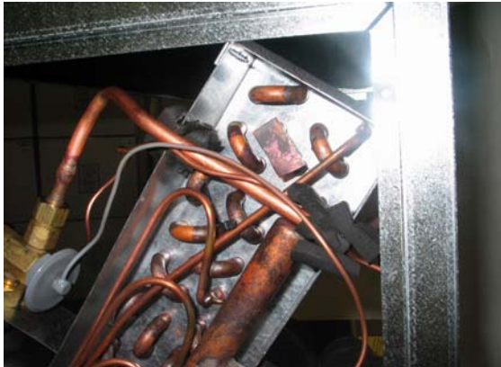
Route both the pressure and temperature tubes as shown.
