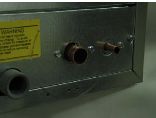
Connection after the end has been cut off.
