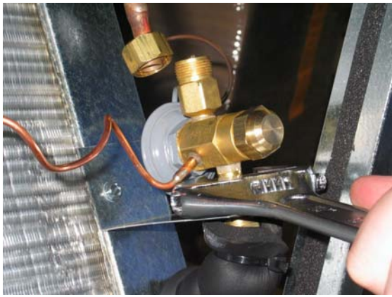
Attach and tighten lower connecting nut as shown.
