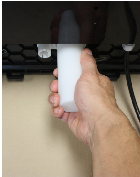
Figure 17: Condensate trap installation
