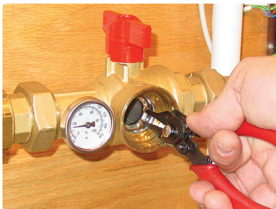
Step 3: Remove the circlip which retains the filter.
