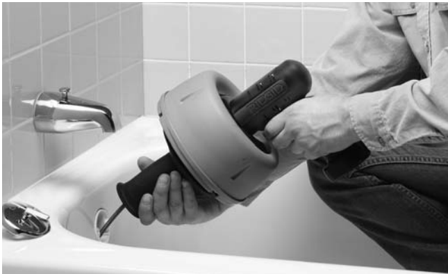
Figure 6 – Push Cable Down Drain Line
